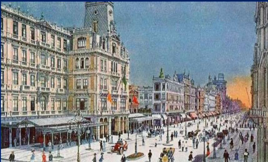
BRÉSIL. — Rio de Janeiro ; Avenue Centrale. Central Avenue. Central Avenue.
